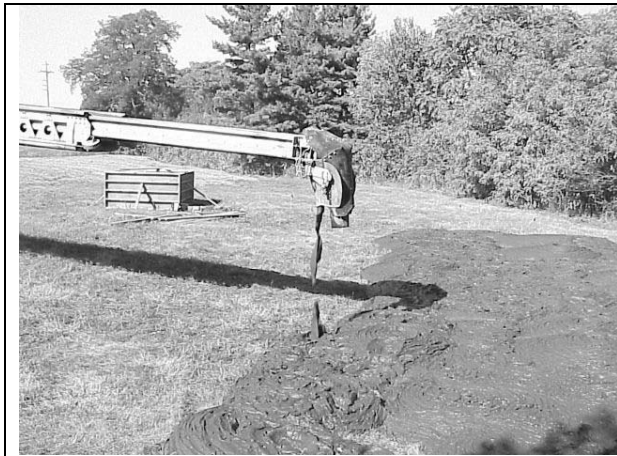
Figure 7. The conveyor boom placed two 20 x 60 foot plots, demonstrating the ability to place sediment at specific depths over a field.
