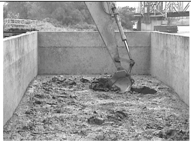
Figure 8. An excavator bucket removing sediment from a barge in Chicago 163 miles from its origin at East Peoria. The sediment was in the barge about a week.
