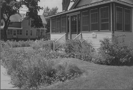
Rain garden, used to filter and treat stormwater from a residence
