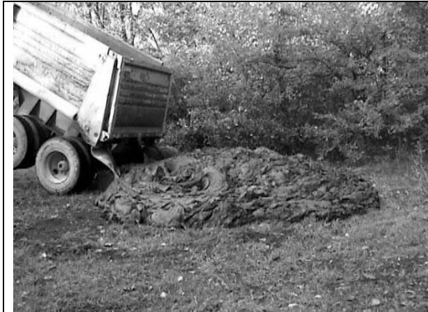
Figure 2. Excavated sediment retains toothpaste like consistency for days when transported by barge or truck. It forms piles when dumped and must dry and weather before developing soil structure.
