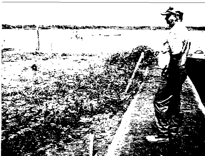
Figure 13. A DNR site manager stands on a geotube in August. The sediment is well consolidated and supports volunteer vegetation. Plants began growing on the island after the first week, but were generally eaten by waterfowl or killed by high water. The geotubes successfully protected the island from erosion during the summer and fall, despite frequent water level fluctuations and high winds.
