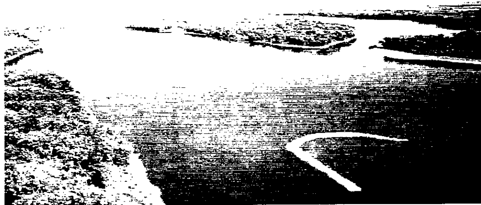
Figure C. Chevron dike field at Mississippi River mile 266. The deep slack water habitat formed behind these structures has been shown to be used extensively by fish in the winter.
