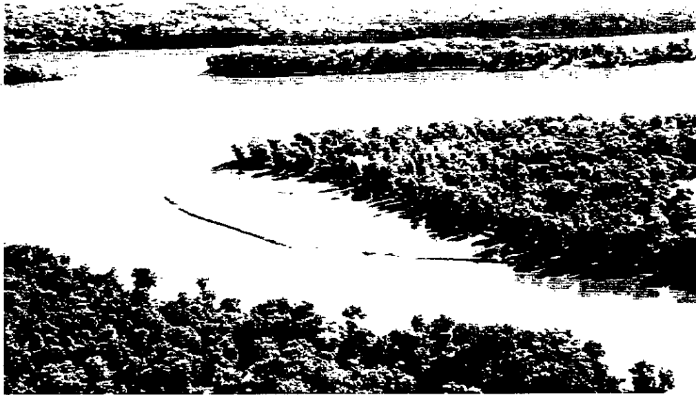
Figure F. Bullnose dike at the head of Peruque Island, Mississippi River mile 235. Note the notch in the structure and the deposition along the head of the island.
