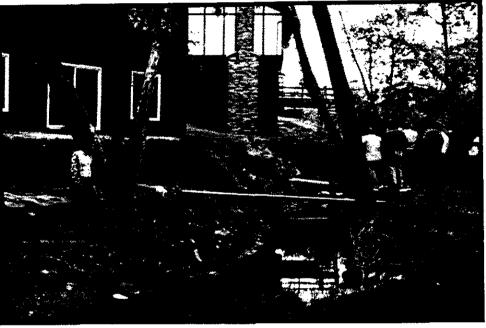
Channel erosion undermined storm sewer and concrete footings of home
