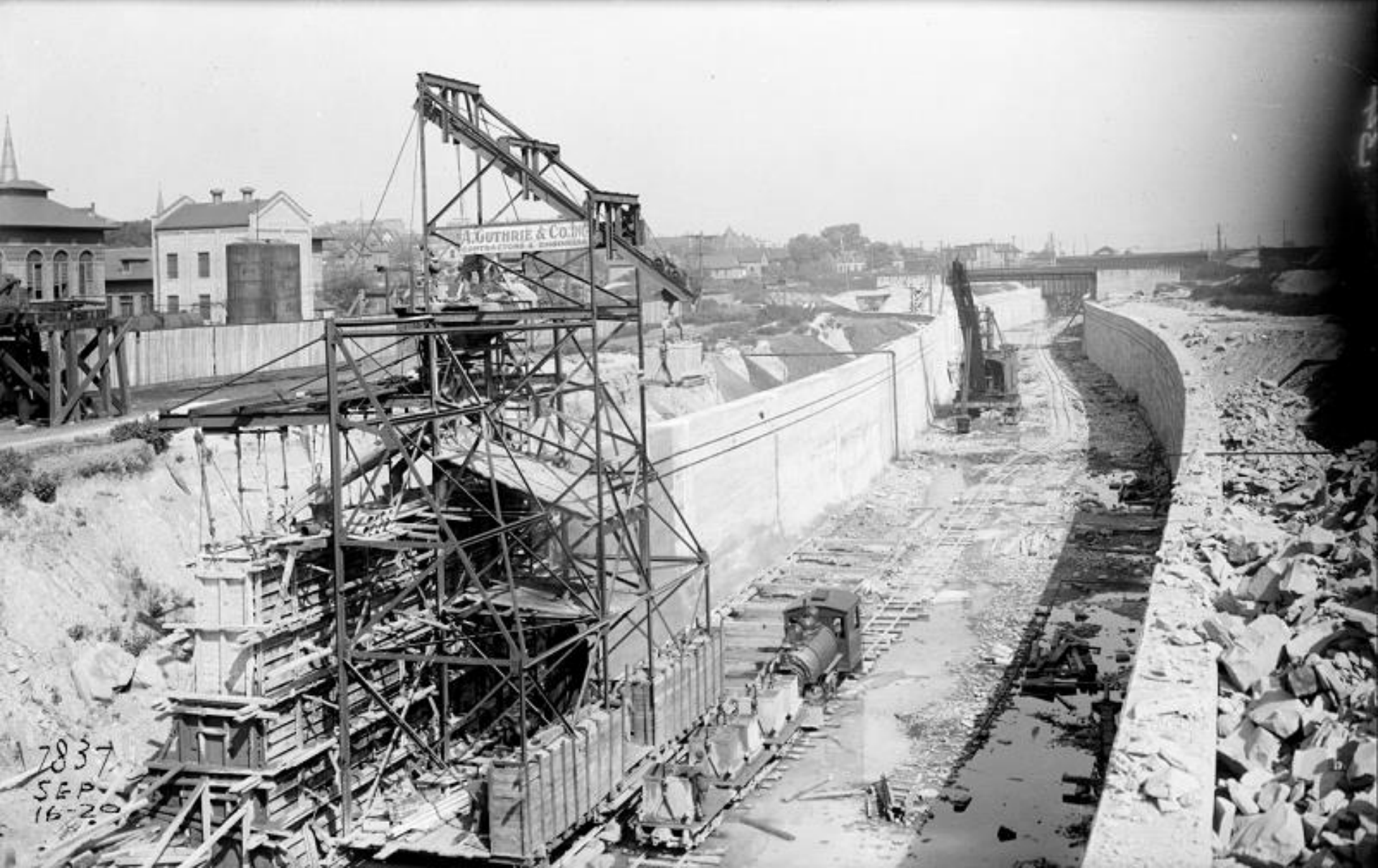
CALUMET-SAG CHANNEL CONSTRUCTED 1911 TO 1922 SIZE IS LIMITED DUE TO LAKE DIVERSION LITIGATION REVERSED THE CALUMET RIVER FLOW
